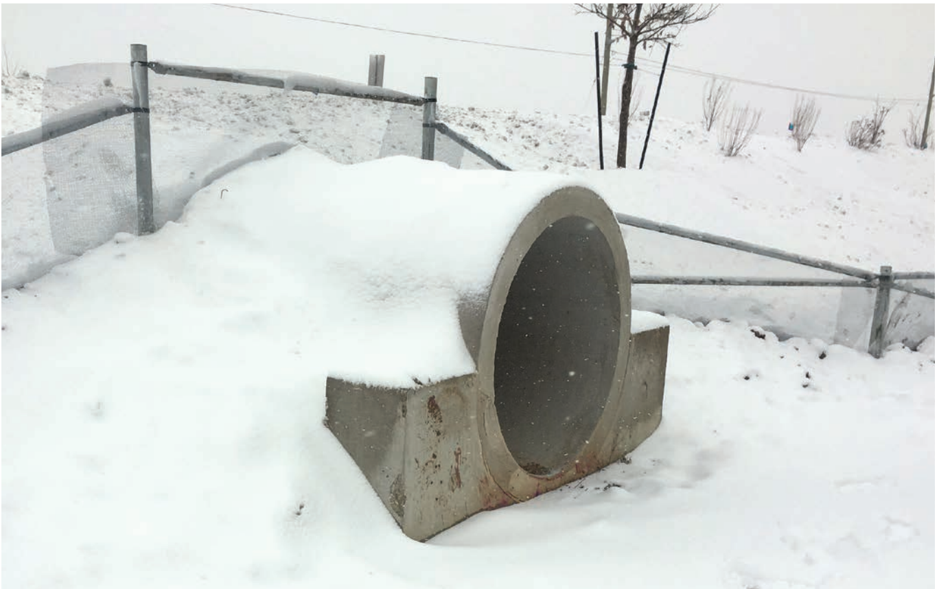
▲ Close up of the Tremaine wildlife crossing. PHOTO COURTESY OF CONSERVATION HALTON.
