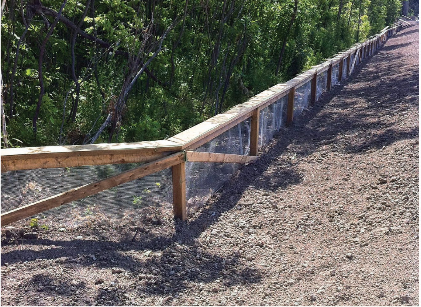
▲ Wildlife fencing was installed during the widening of Neyagawa Road in Oakville, to direct small animals to a safe crossing. PHOTO COURTESY OF CONSERVATION HALTON.
